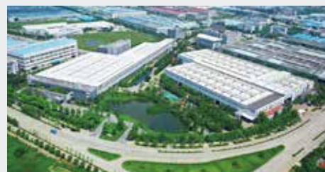
China Gaoli Headquarter and Factory
